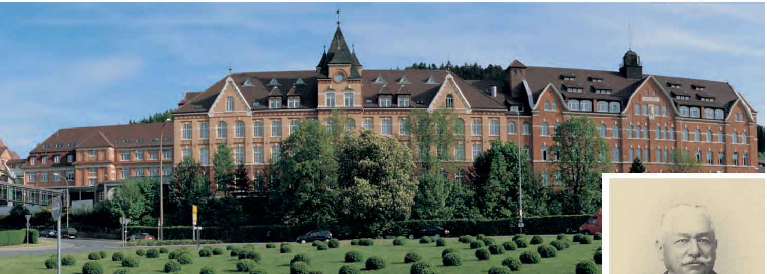
Aesculap AG World Headquarters in Tuttlingen, Germany
